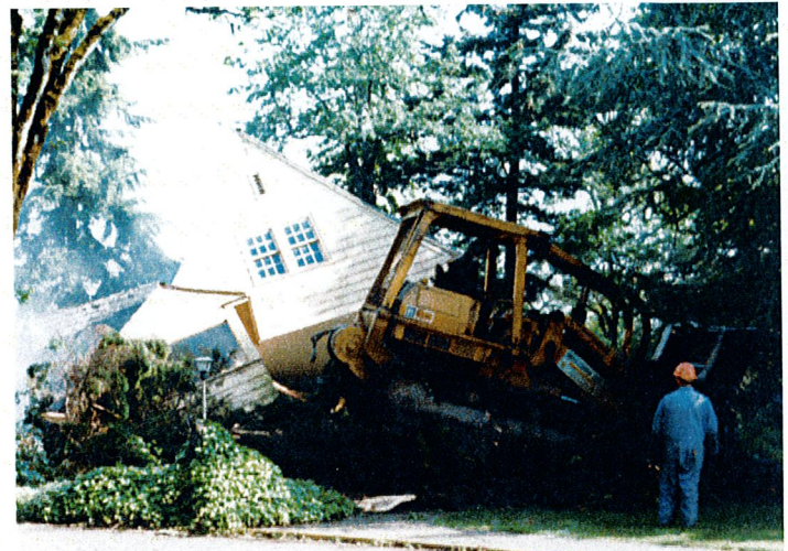
Manse/Harris Hall Demolished - May 1986
