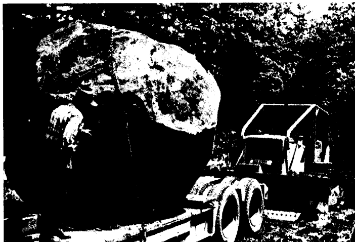
Removing boulders for new addition - 1960
