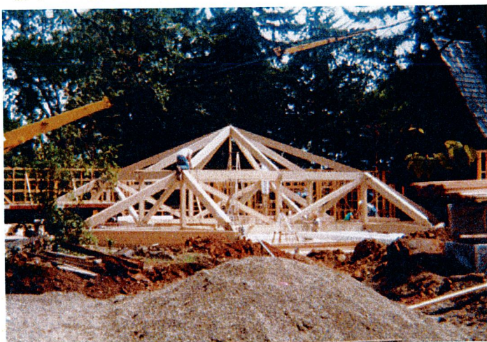
New Sanctuary Roof Truss - October 1986
